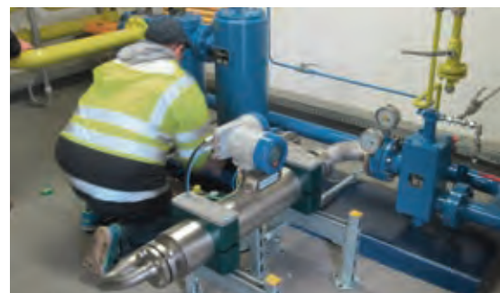
MID MI-005 tanker filling system for liquefied gas
